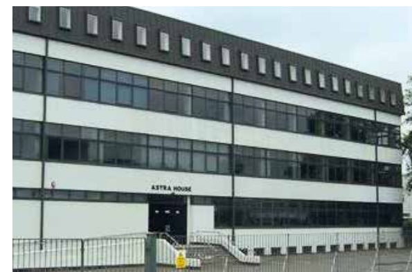
Astra House, Harlow
